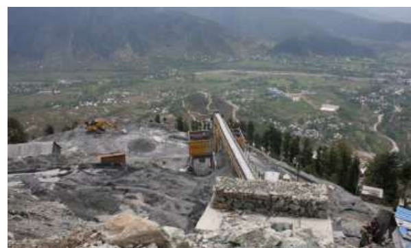
Work in progress on the Kishen Ganga Hydro Electric Power Project in North Kashmir district of Bandipora in 2012. NISSAR AHMAD
