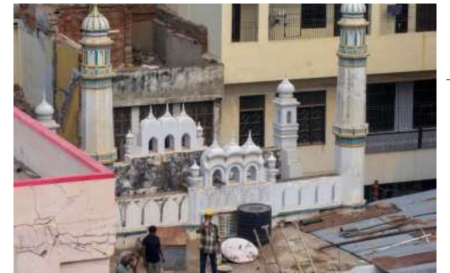
Workers demolish a portion of the Mirza Karimullah Beg Mosque during a road-widening drive in Varanasi on Wednesday. PTI
