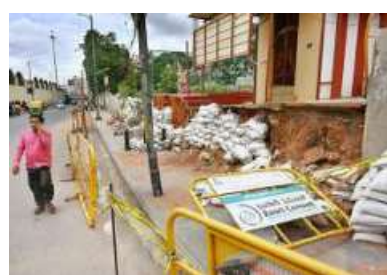
The aftermath: The area around Bowring and Lady Curzon Hospital has been restricted following the wall collapse. ALLEN EGENUSE J.
