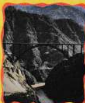
Chenab Rail Bridge : p. 10
