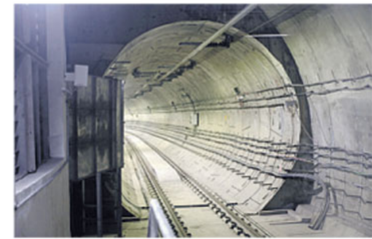
The Kalbadevi Metro station on Tuesday
