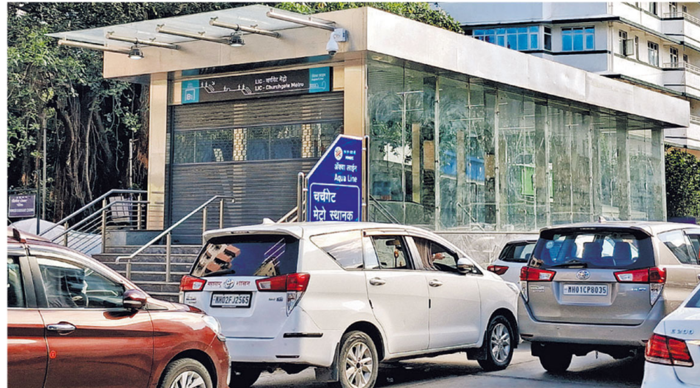
Churchgate Metro station, part of the new Aqua Line 3 corridor. PIC/RAJENDRA B AKLEKAR
