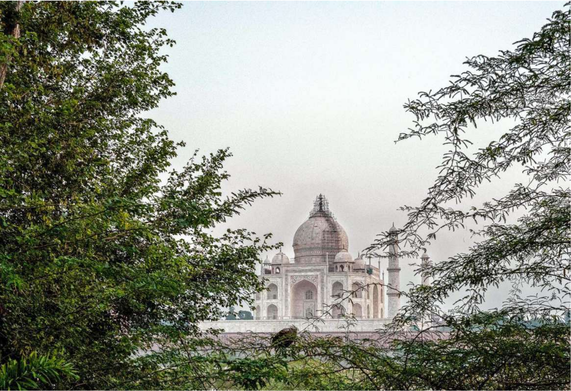
Surreal beauty: Scaffoldings are put up as restoration work goes on at the dome of the Taj Mahal in Agra on October 17. AFP
