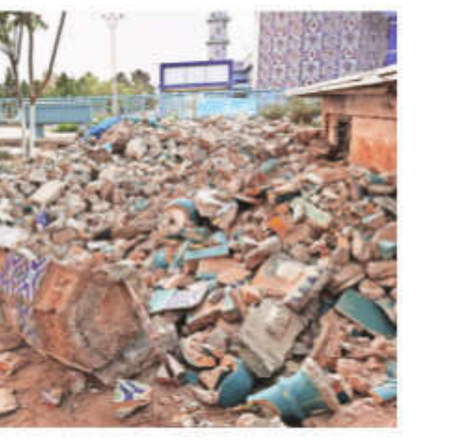
Damage is seen in the historic Blue Mosque in Mazar-e Sharif after the quake on Monday. AP
