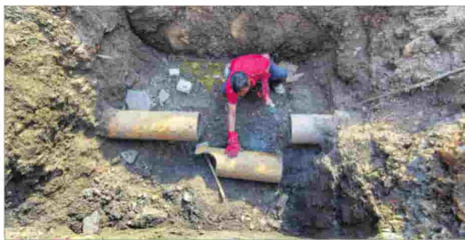
SMART CITY: Restoration work of water pipelines after the water contamination tragedy in Indore, M
