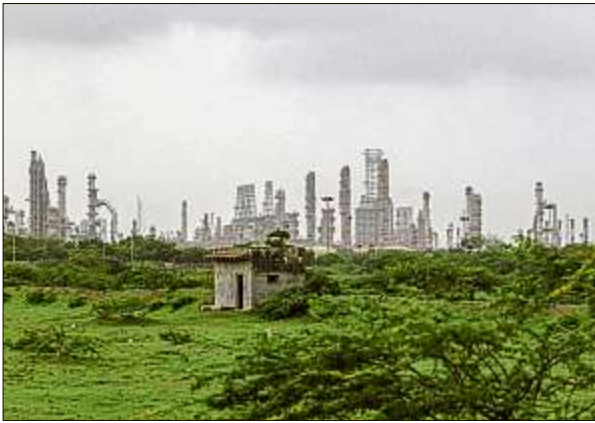
Reliance's Jamnagar refinery complex.
