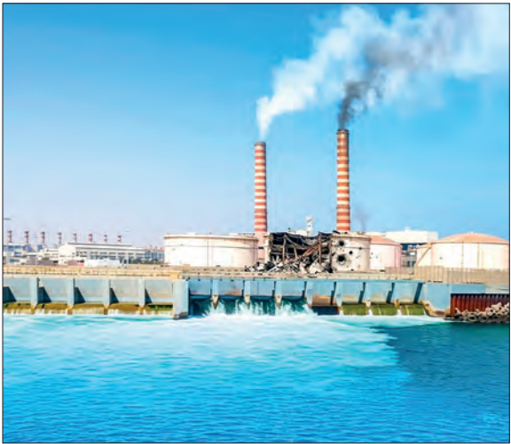
An Iranian attack struck a power generation and water desalination plant, causing extensive damage to the facility. PHOTO: NEWS OF BAHRAIN/FACEBOOK
