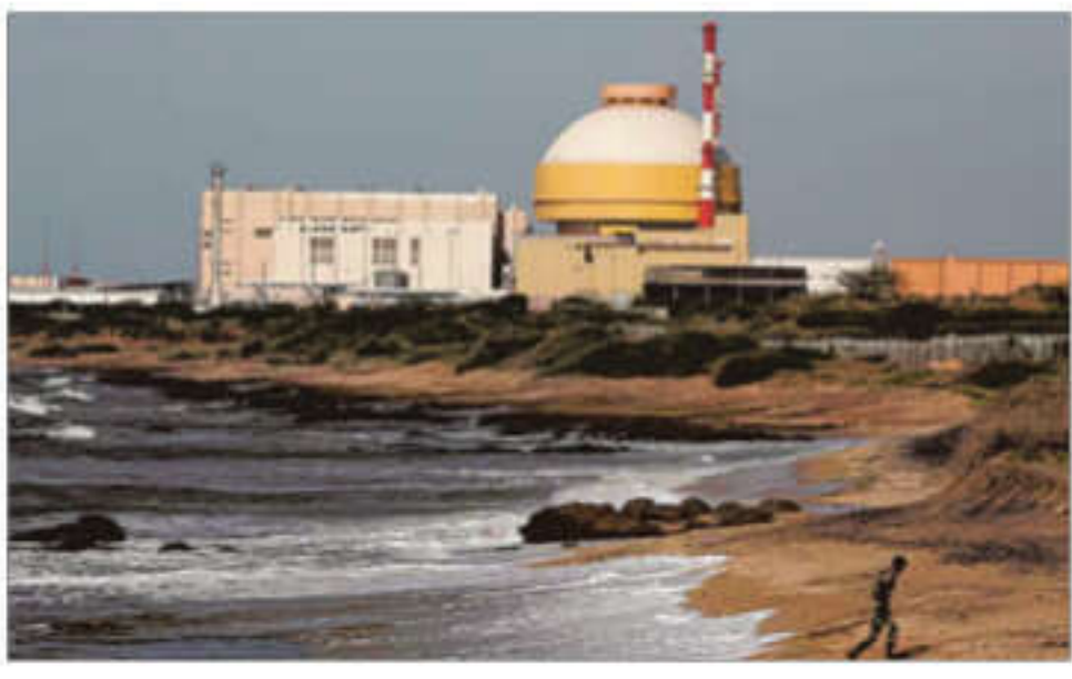
The Nuclear Power Corporation of India Ltd (NPCIL), which operates the plant, has downplayed the recent leak. REUTERS
