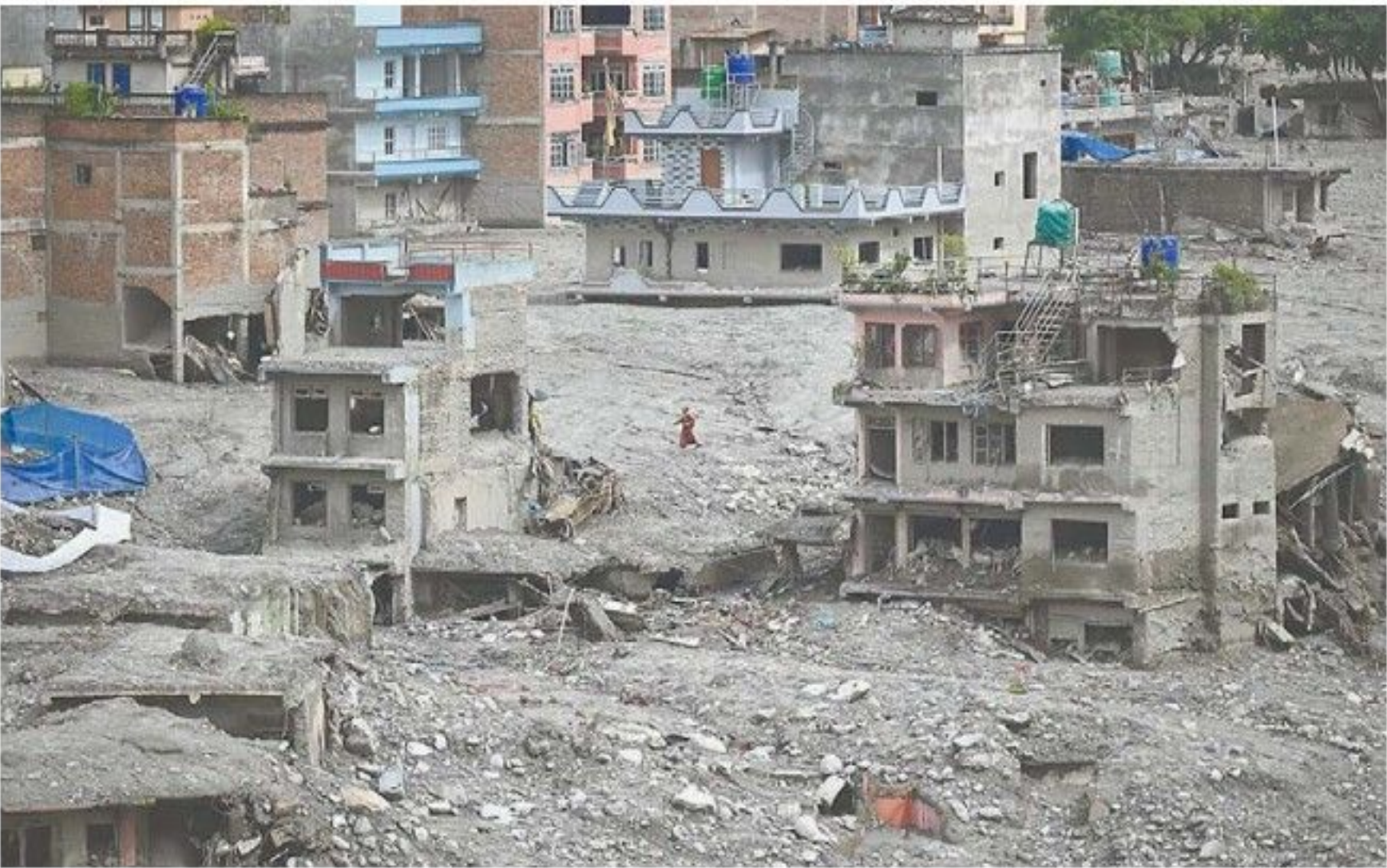
Houses damaged by last month's massive flash floods in the town of Trishuli in Nepal's Nuwakot district on Friday AFP-JJII
