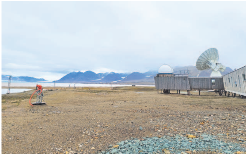
(top) The Ny-Ålesund railway on Spitsbergen, Svalbard, which operated from 1917-62; rapidly rising temperatures are melting permafrost and destabilising existing structures.
