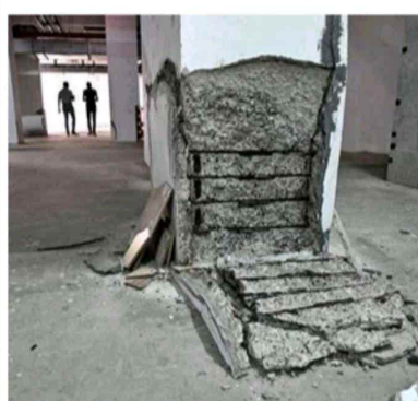
Constant threat: (clockwise from top) A building material caught on a safety net tied around the twin towers of Chander Kunj Army Towers to prevent debris from falling on people underneath; chunks of concrete have fallen off the roof at many places in the towers; a foundation pillar stripped off concrete exposing the rusted reinforcing bars. THULASI KAKKAT
