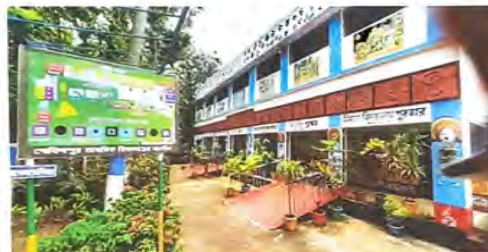
The present school building
